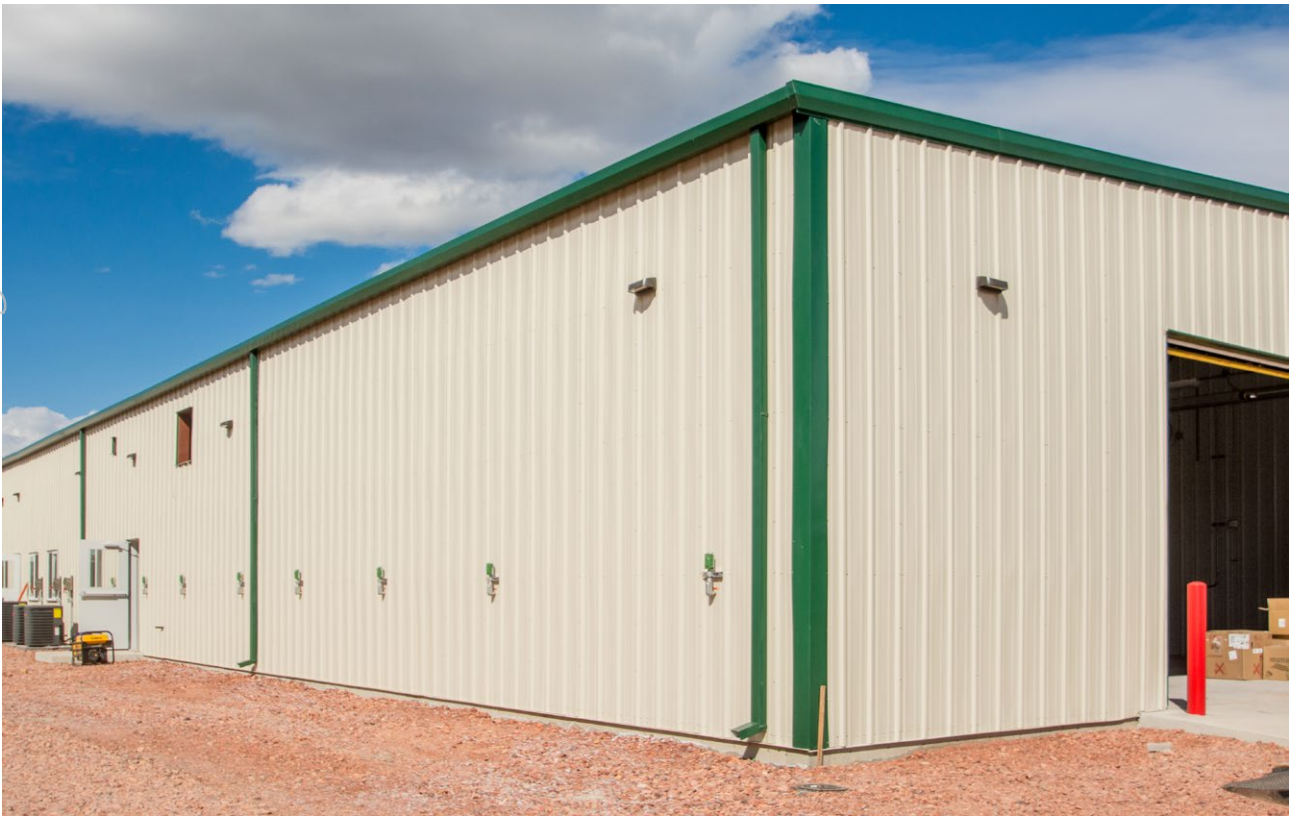
Figure 2: Administration and Workshop Building, Wyoming, USA
