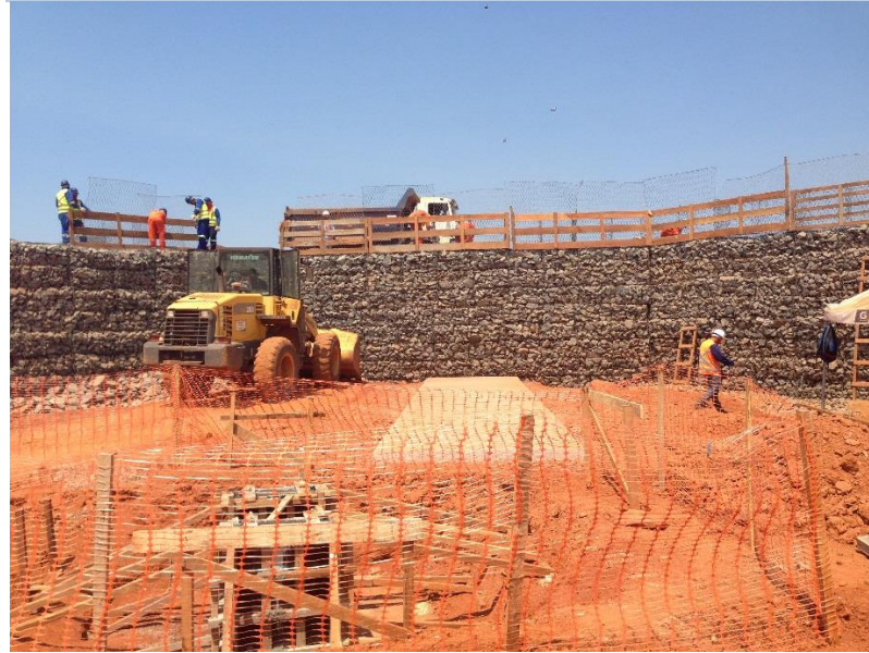
Fig. 2: Antas project crusher civil works
