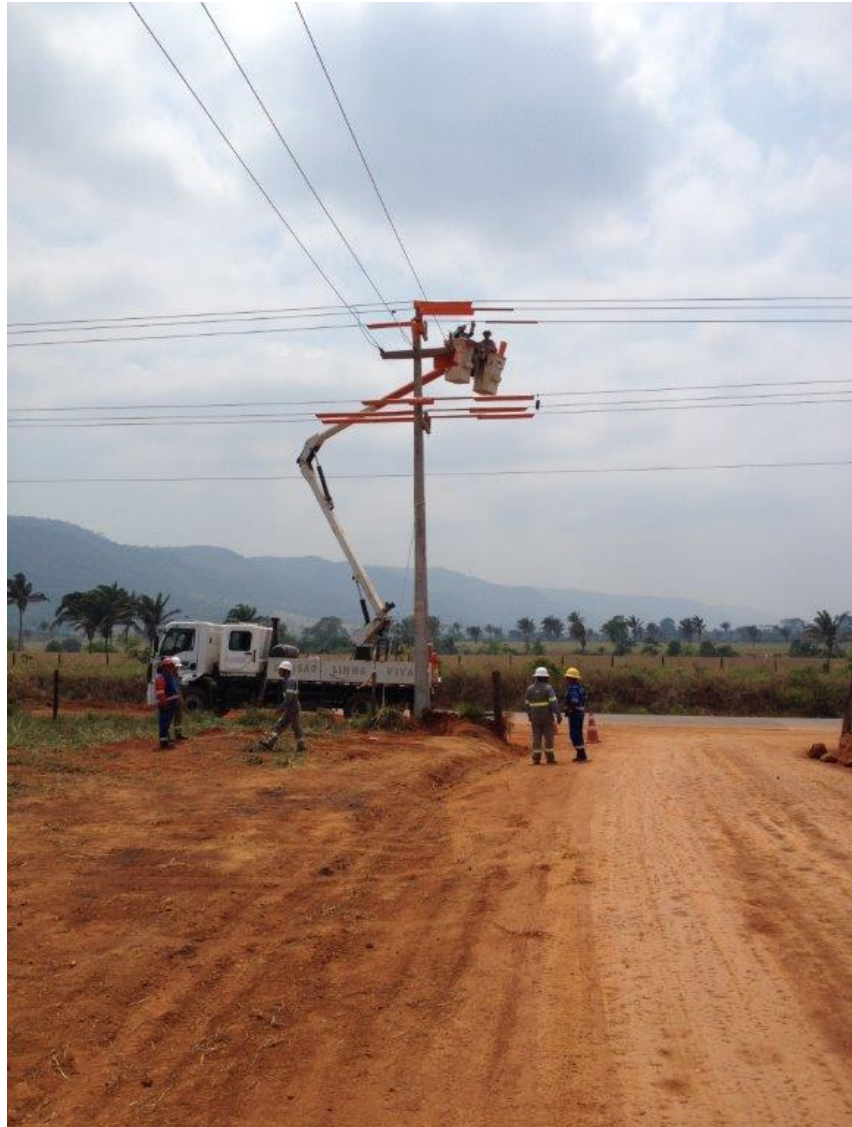
34.5Kv power cables being connected to the transmission poles
