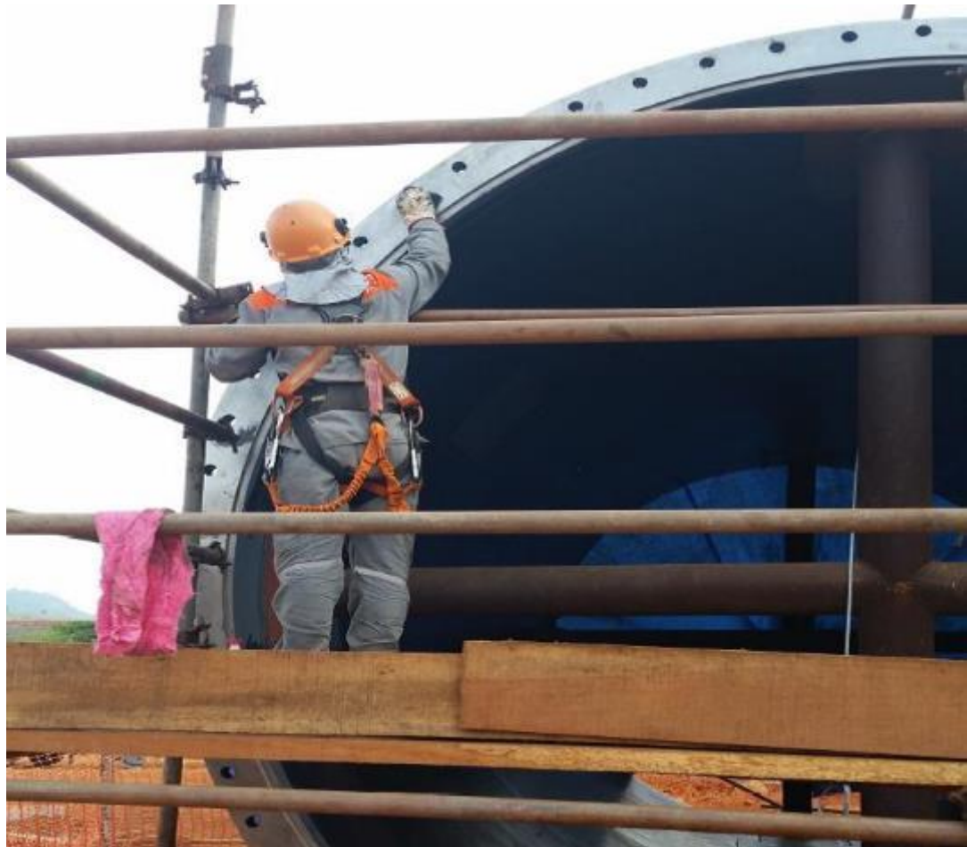
The 12'x24' Metso Ball Mill shell (flanges) being prepared for mounting of the trunnion heads
