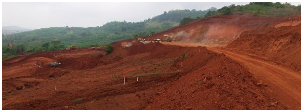
Establishment of mining benches - Antas Stage One
