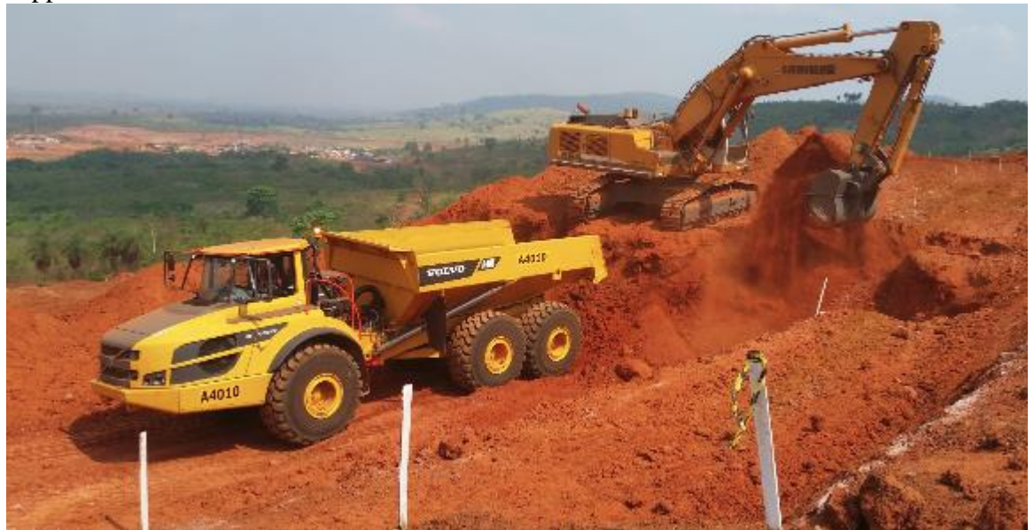
First loads - Volvo A40F and R964 excavator
