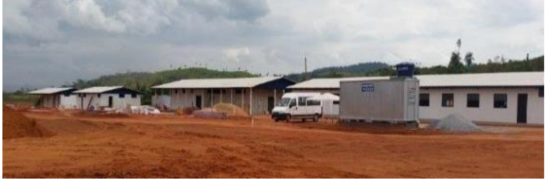
Administration offices, dining hall and first aid post, all well advanced
