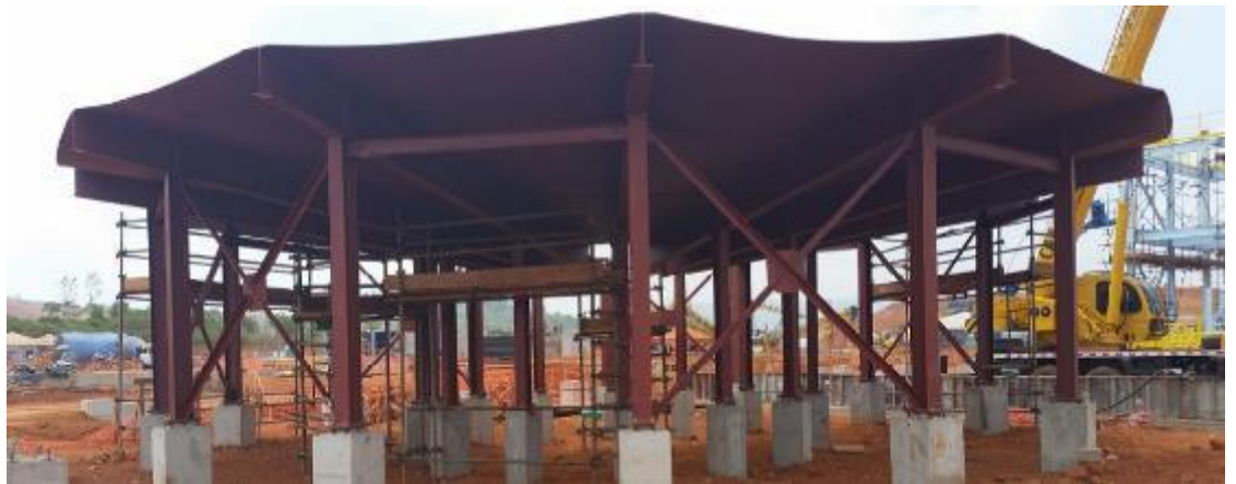
Concentrate Thickener fabrication in progress
