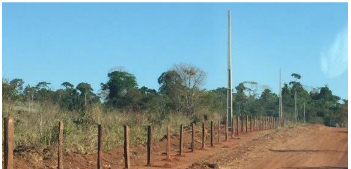
100 pylons have been installed in readiness for suspending the 34.5 kV transmission line
