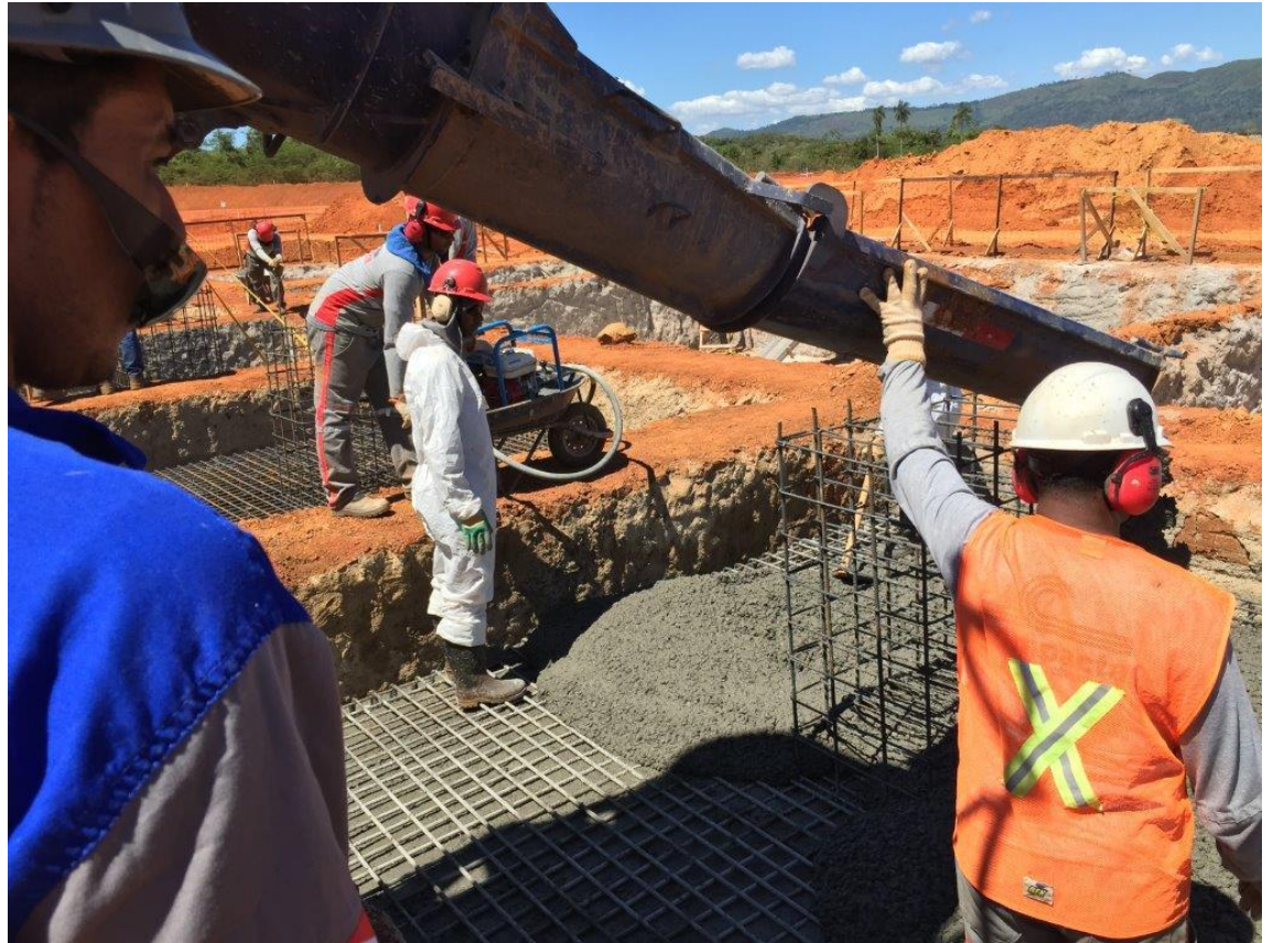
Pouring of Concrete
