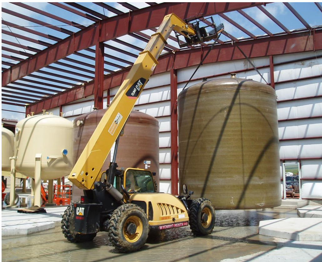
Figure 2: Setting fibreglass tanks inside the CPP
