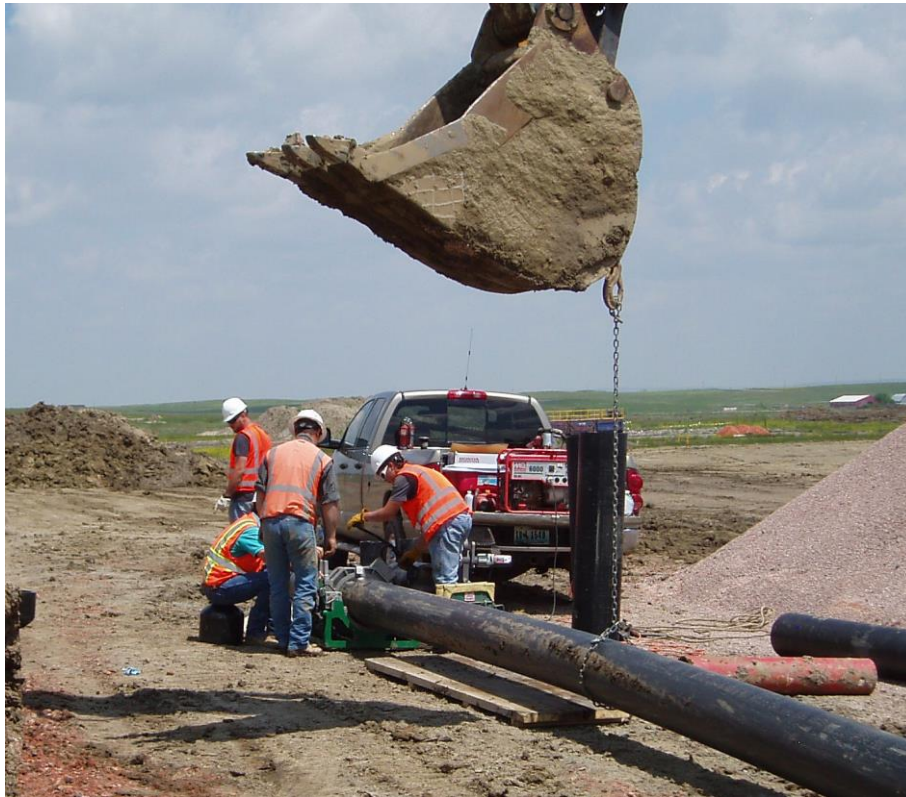
Figure 3: Pipe laying in Mine Unit 1
