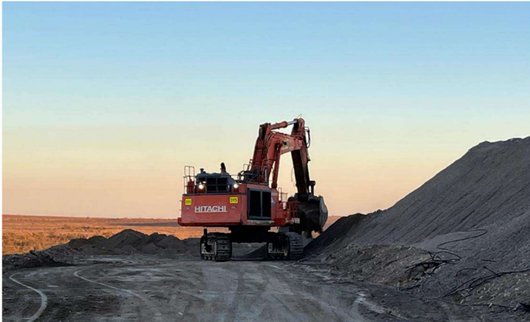
Figure 3: The recently mobilised 120T excavator working on northern berm of Heap Leach pad
