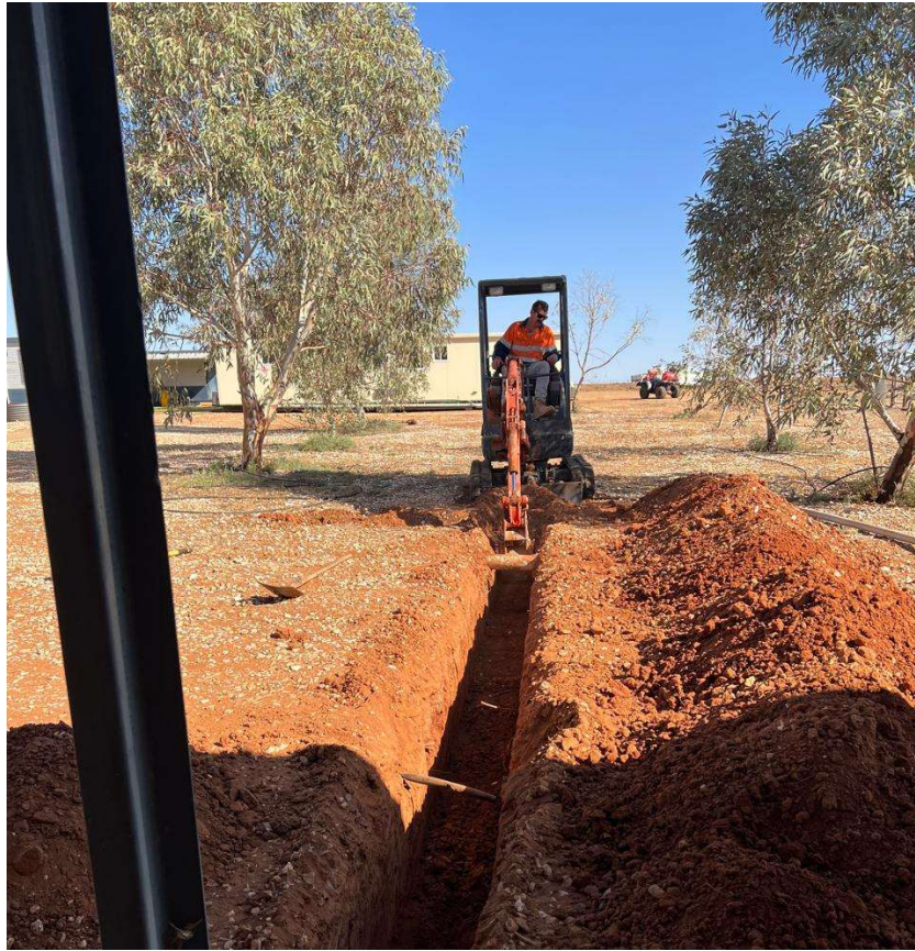
Figure 3; Camp expansion underway with 3 additional units being installed
