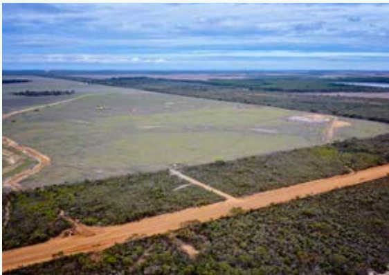
Figure 7. Aerial view of the Springdale Graphite Project site.
