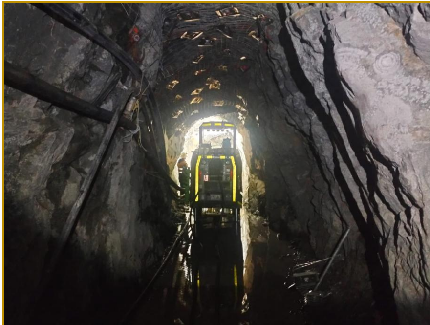
Figure 2 New Epiroc TD1 Jumbo at work in the Amalgamated Adit
