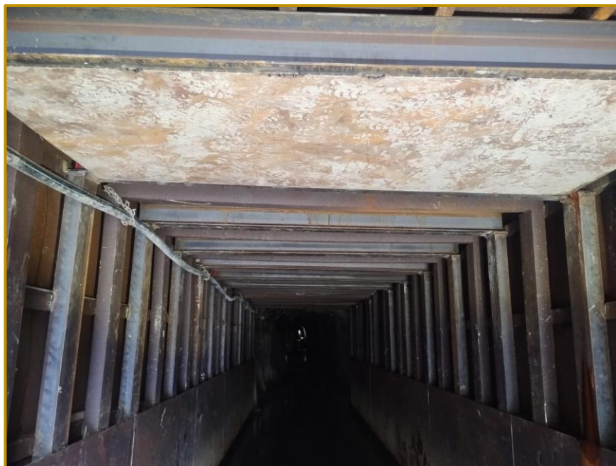
Figure 8 New steel sets installed to reinforce the Portal structure into the Reward Mine.
