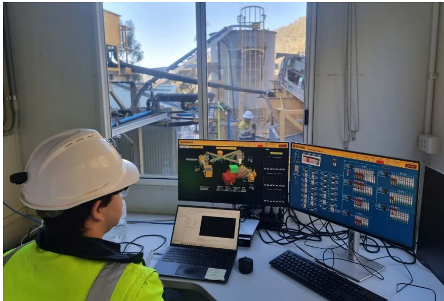
Figure 8: Automation programming technician testing the Reward gravity plant systems from control room
