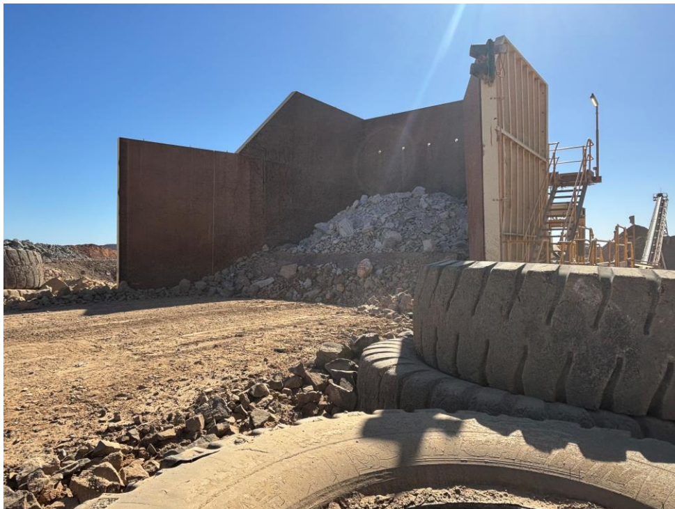
Figure 1 - First bucket of Brightstar ore loaded into the crusher at the Laverton Mill
