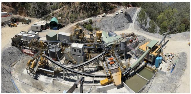
Figure 5 Birds eye view of the Hill End Gravity Gold plant with sorter (left side)
