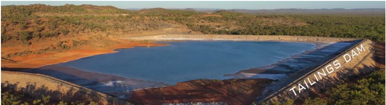
Figure 7. Mungana tailings dam.
