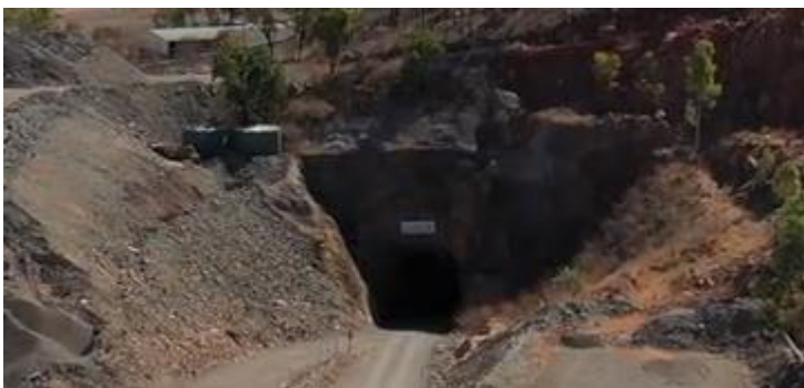
Figure 6. Mungana underground portal (Source: Auctus Resources)
