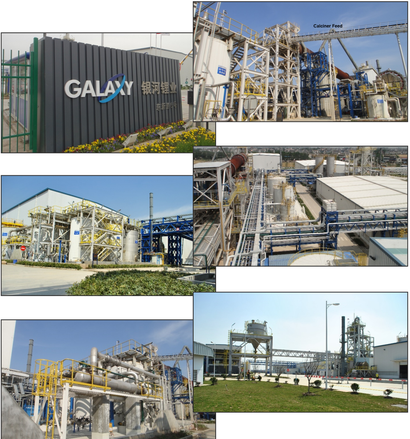
Figure 6: Galaxy Jiangsu Lithium Carbonate Plant
