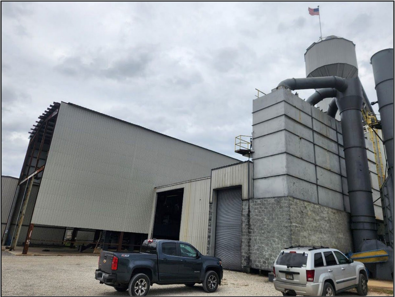
Figure 1: Front view of the Kentucky Plant, highlighting its conversion to a high-capacity Activate Carbon production facility
