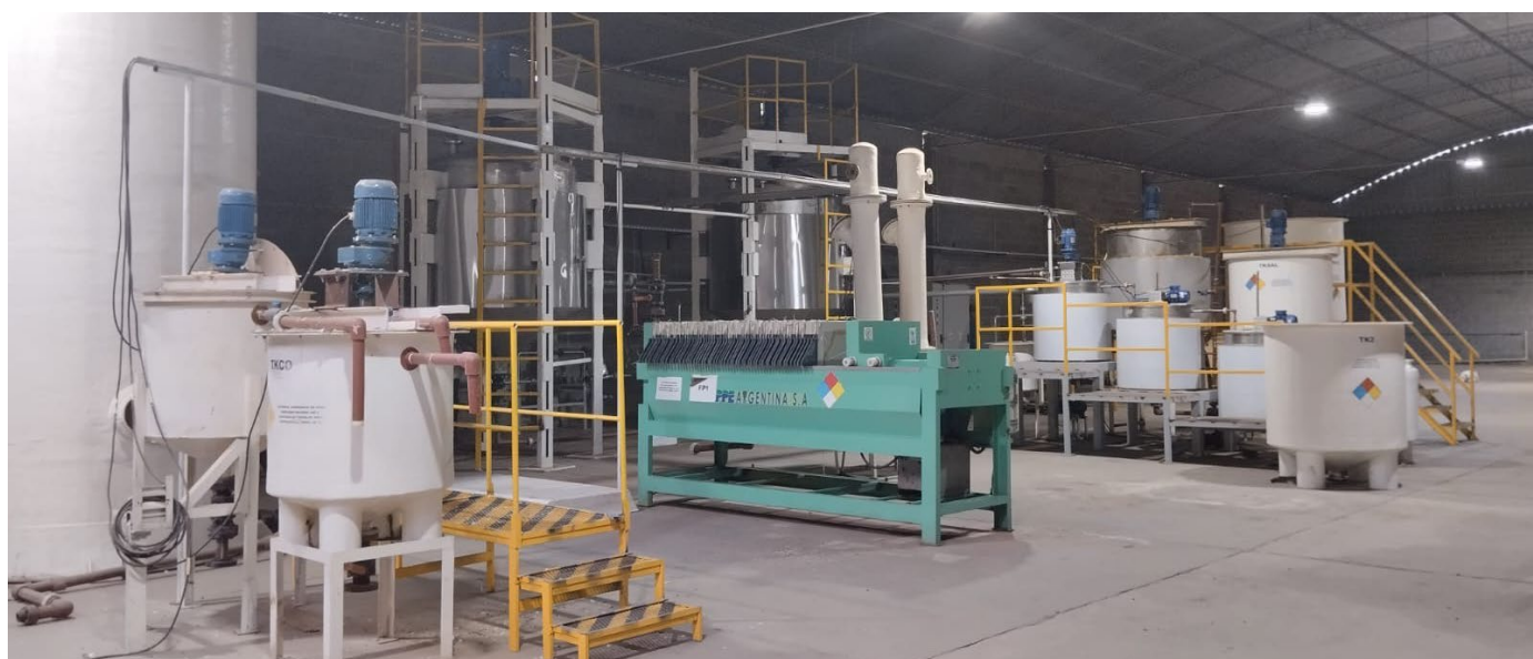
Figure 5: 250tpa Lithium Carbonate Plant at Pursuit's purpose facility in Salta, Argentina
