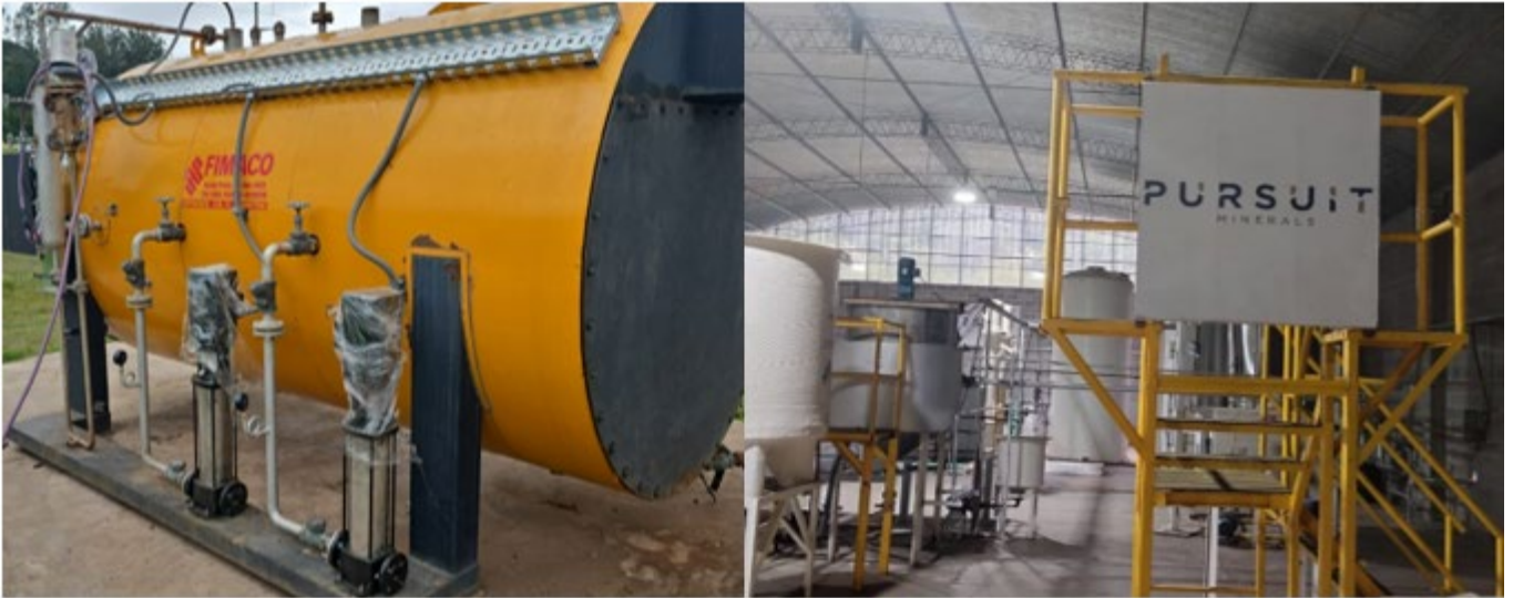
Figure 6: Boiler installation at the 250tpa Lithium Carbonate Plant in Salta.
