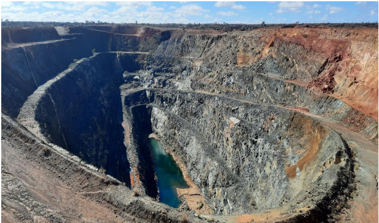
Figure 6: Existing Fish open pit
