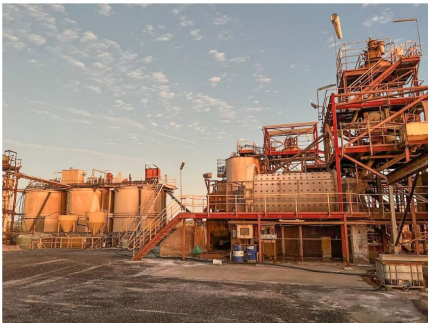
Figure 2 – Lorena Processing Facility
