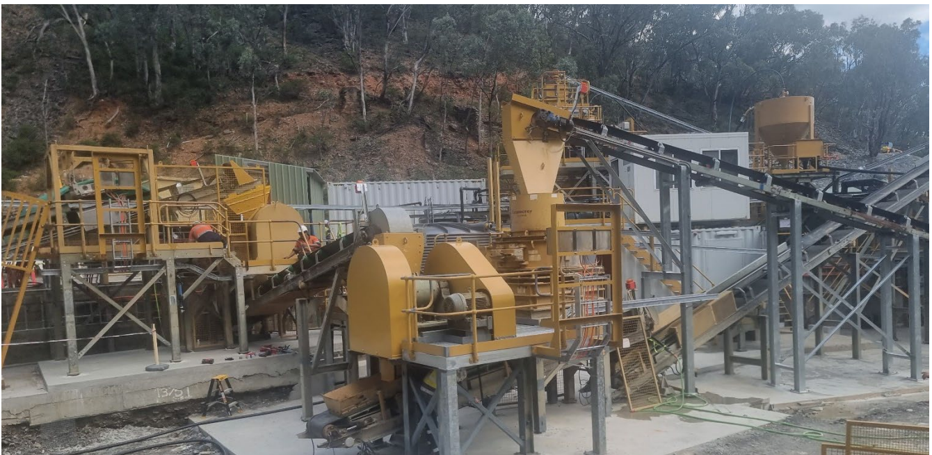
Figure 5 Reward gravity gold plant looking over the 2 jaw crushers and the impact crusher.
