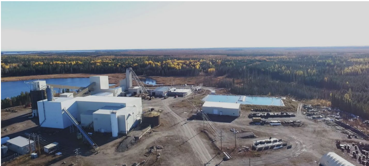
Figure 1: Wabowden Project - Bucko Mine and Processing Facility
