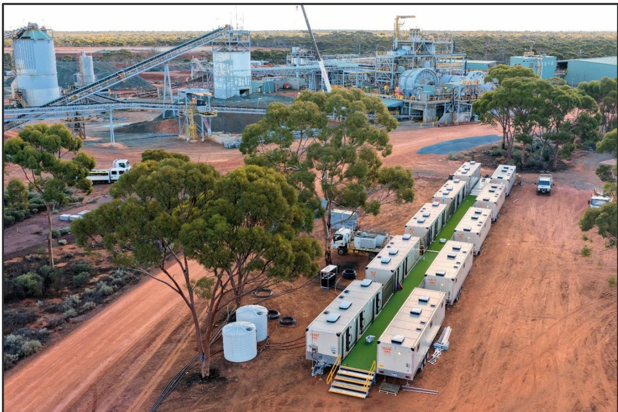
Figure 3 – BSHP Construction Camp Stage 1
