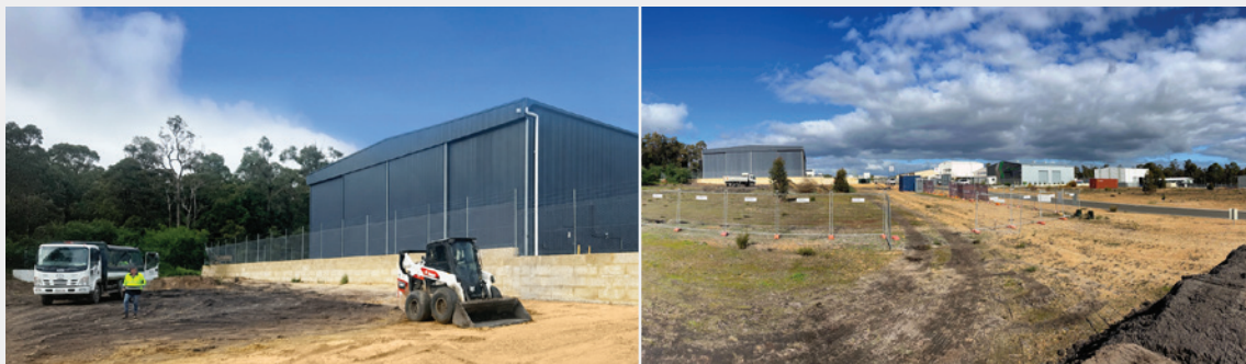
Figure 2. Earthworks underway for the new Collie Micronising Facility.
