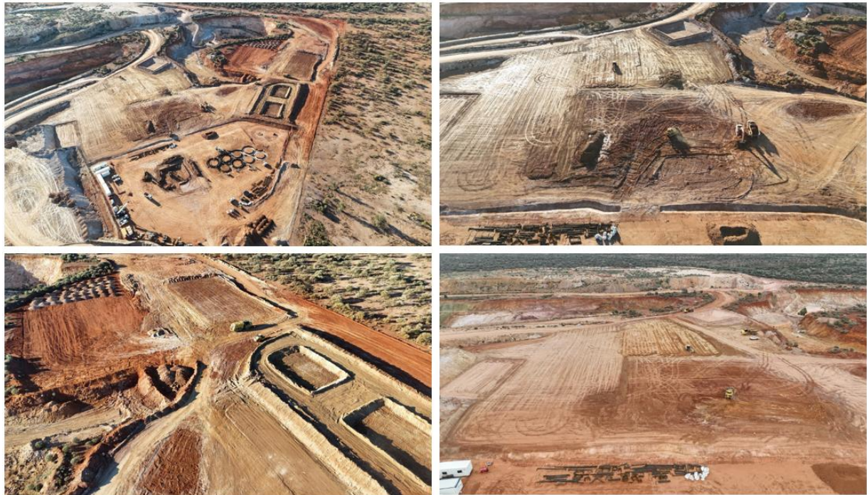
Figure 3 - Construction activities underway (June 2026, post-FID )
