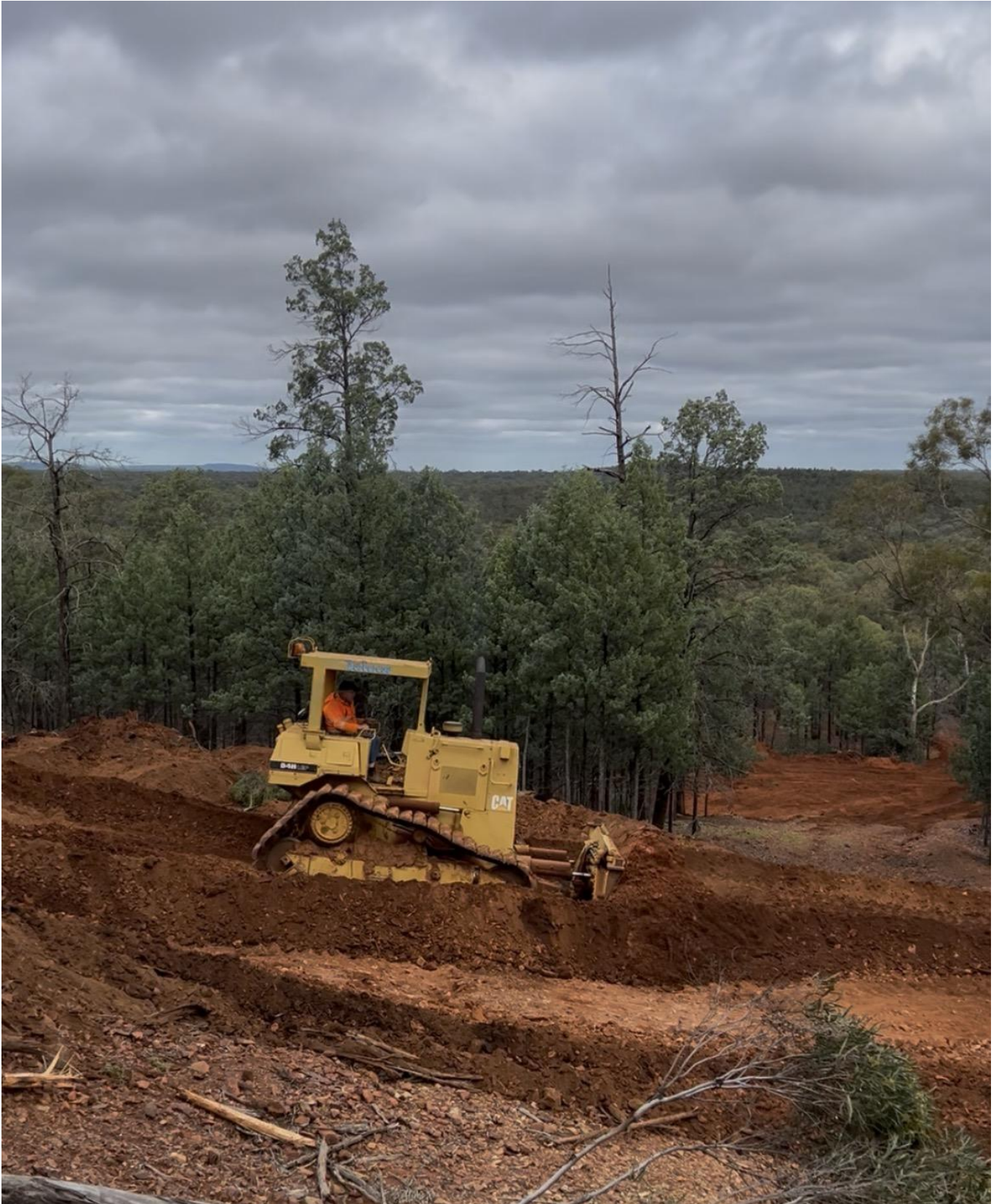
Figure 2: Mt Solitary drill pad/track construction
