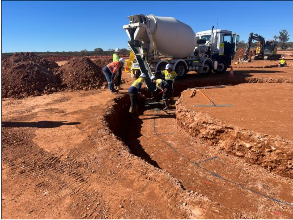
Figure 3 - First concrete being poured for CIL tanks (24 June 2026)
