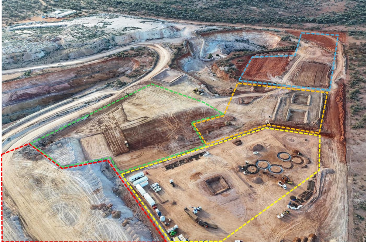
Figure 1 - Earthworks and first concrete poured for CIL tanks (28 June 2026)
