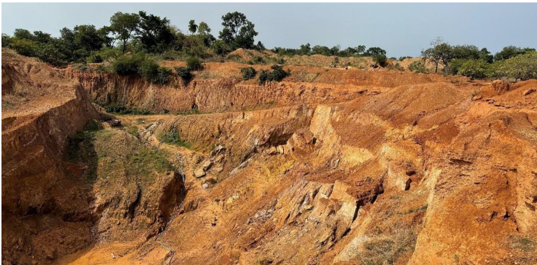
Figure 8: Failure on BMT1 west wall
