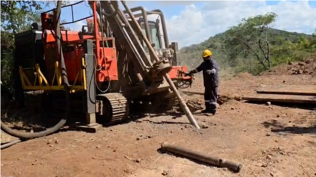
Figure 2 – Commencing drilling on the first Tundulu hole
