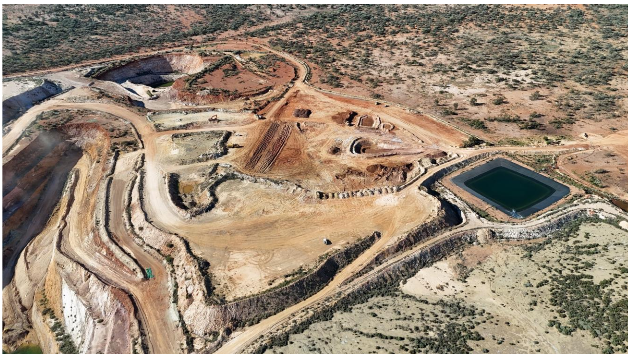
Figure 2 - Site remediation works underway in preparation for construction to commence
