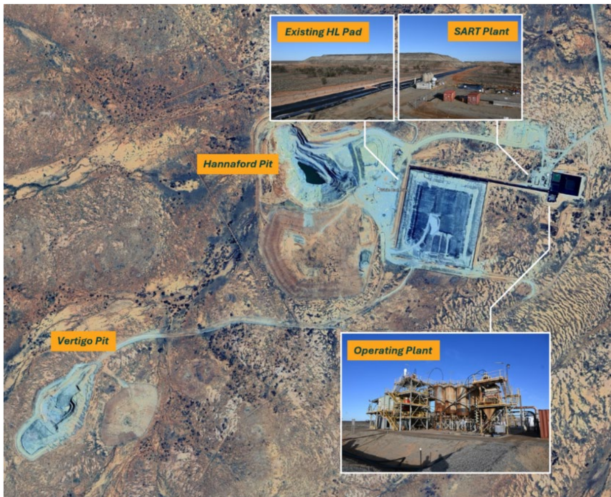
Figure 2: Aerial view of White Dam gold operations site with photos of existing operating infrastructure and heap leach pad
