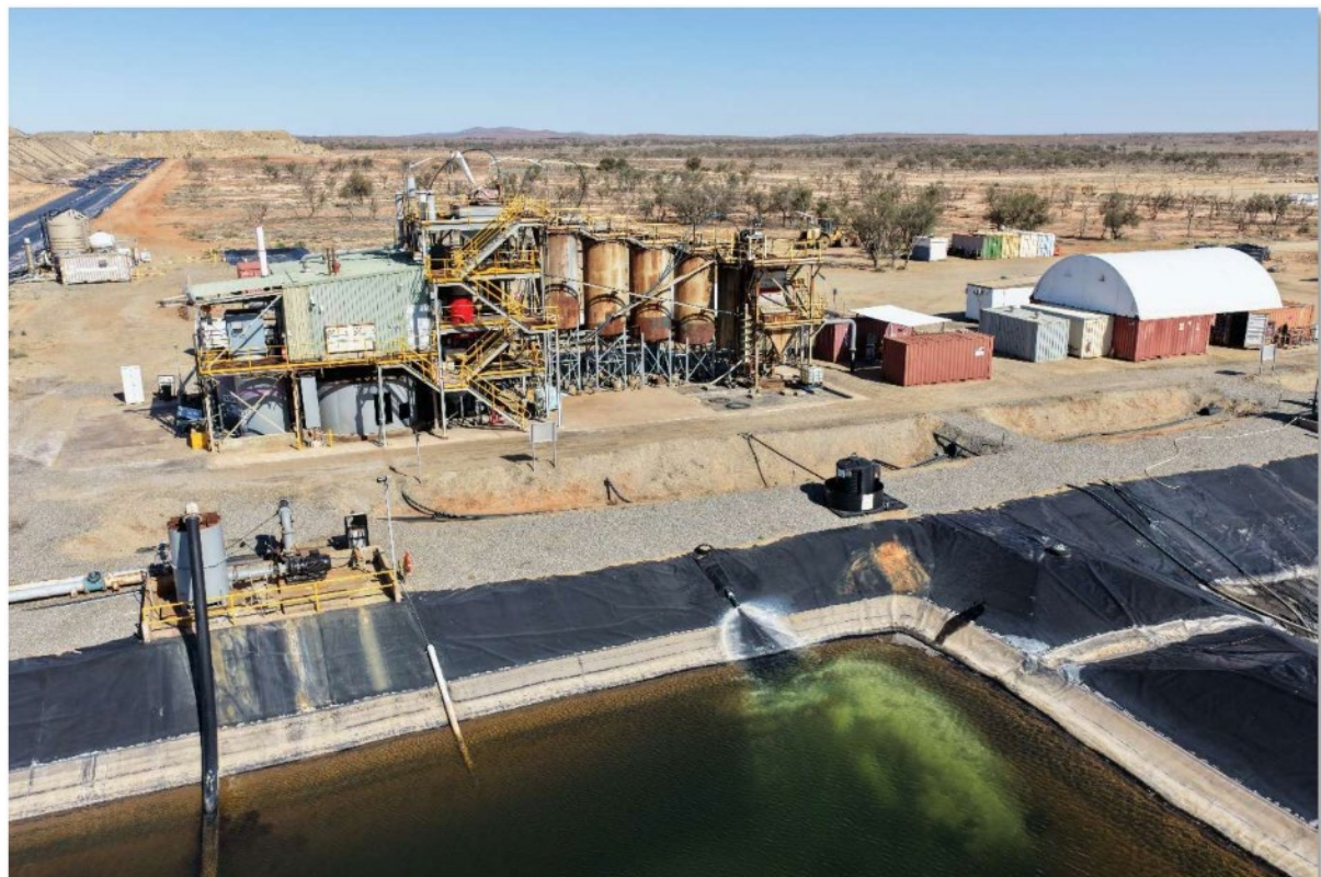
Photo 2: Aerial view of Plant now fully approved and operational
