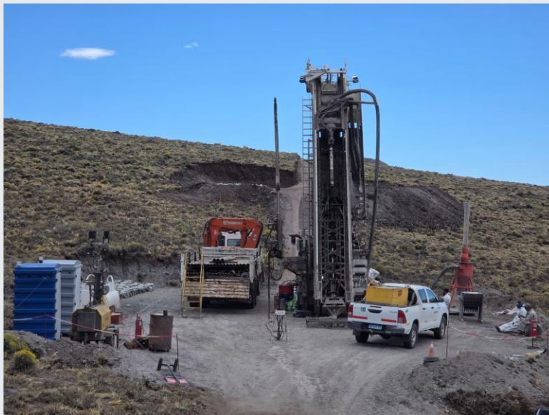
Figure 1: Reverse circulation drilling at the Cerro Chacón Gold Project (CGRC034).
