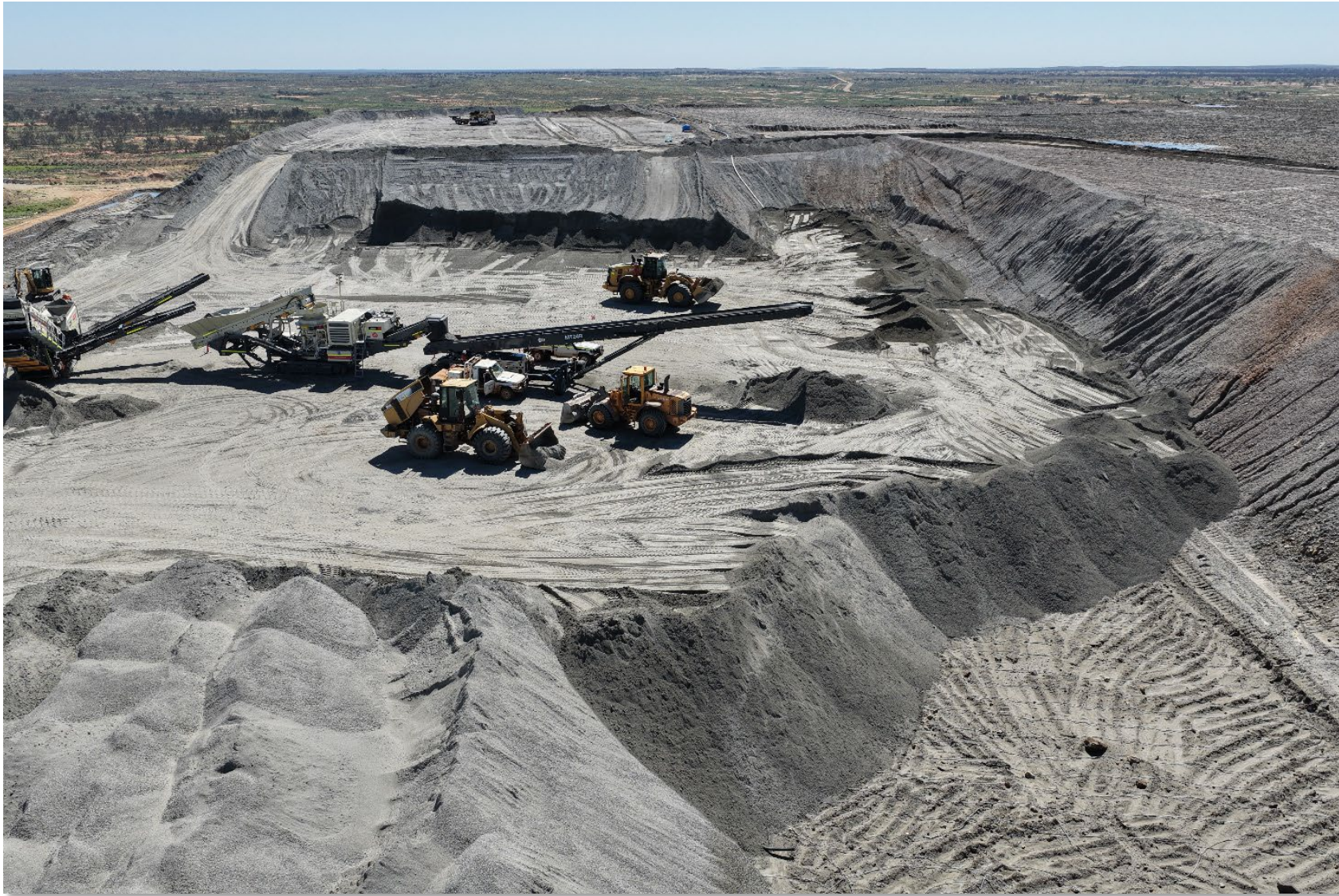
Photo 3: Re-crushing circuit in operation in south western corner of final pad lift
