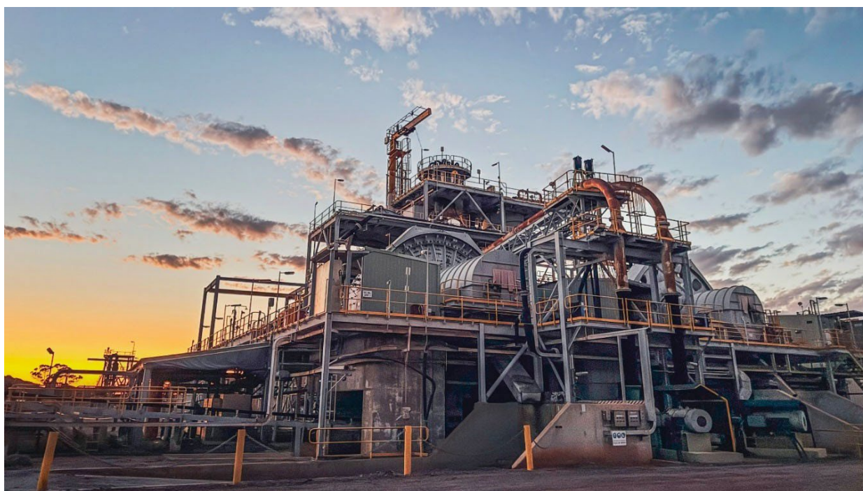
Figure 4: Black Swan Project – Existing SAG & Ball Mills
