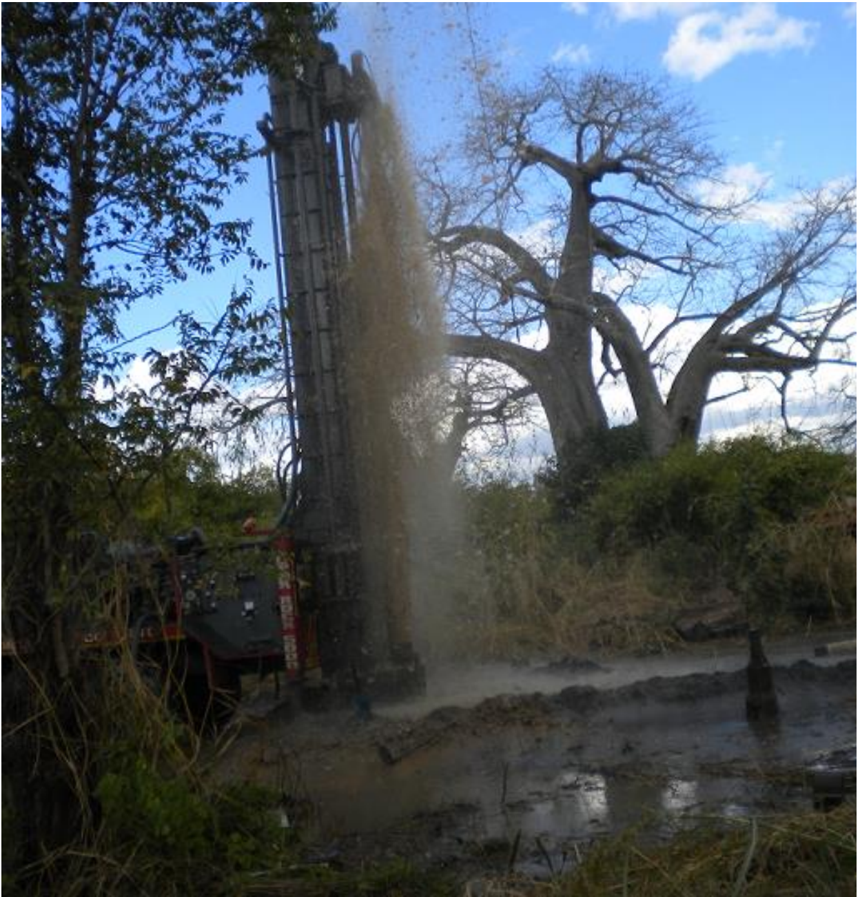
Figure 3 – Recently completed Water Bore Hole
