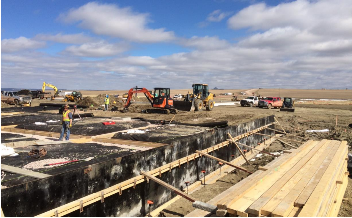
Figure 1: Form work for CPP foundations
