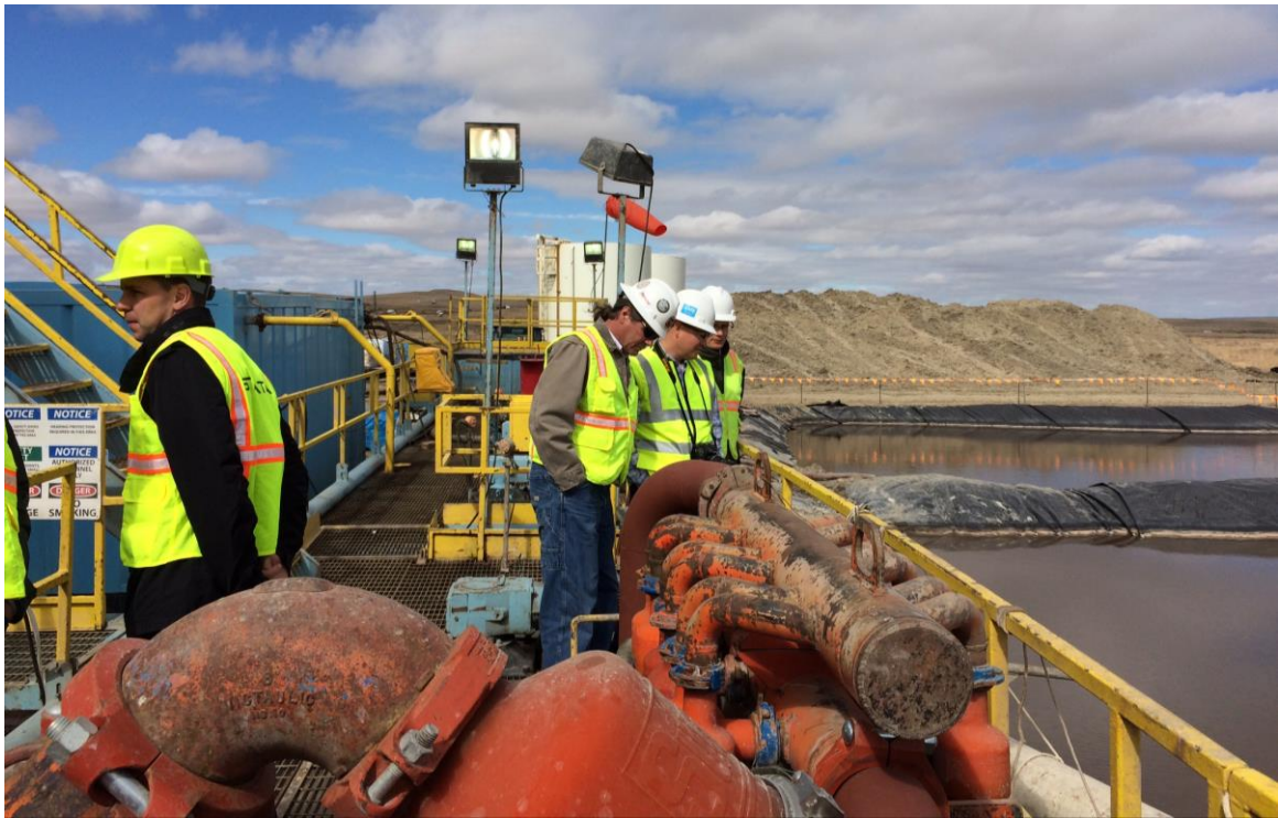
Figure 5: Deep disposal well drill rig platform
