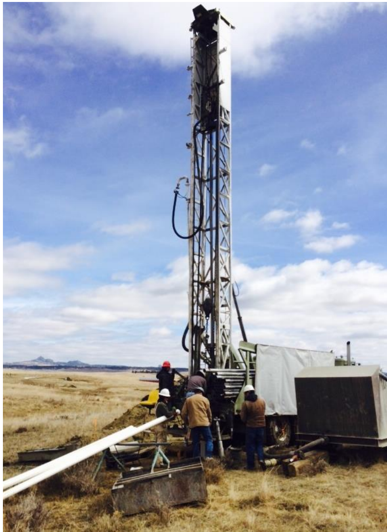
Figures 7 & 8: Drilling of monitor and mining wells
