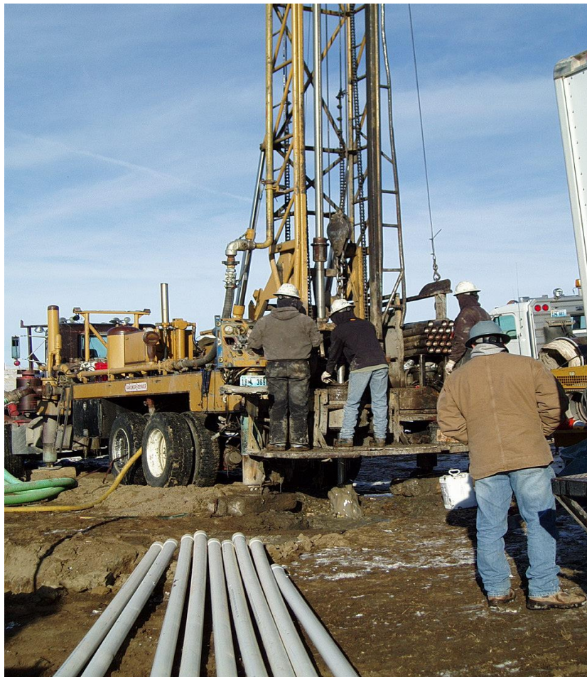
Figure 6: Drilling of monitor and mining wells
