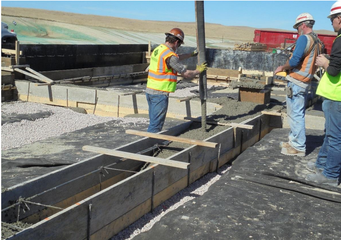
Figure 2: Pouring of foundations for CPP
