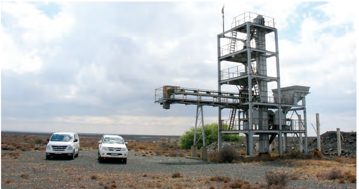
The trial mining processing facility is 30km from the township of Beaufort West which has a population of 30,000 people
