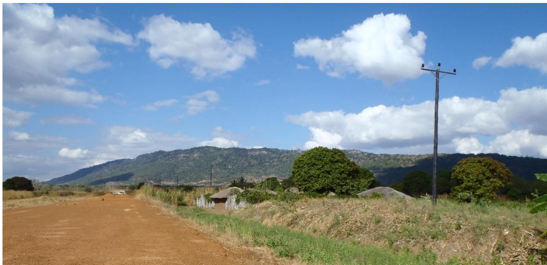
Figure 6 – Power lines being installed along the road from MontePuez to Balama
